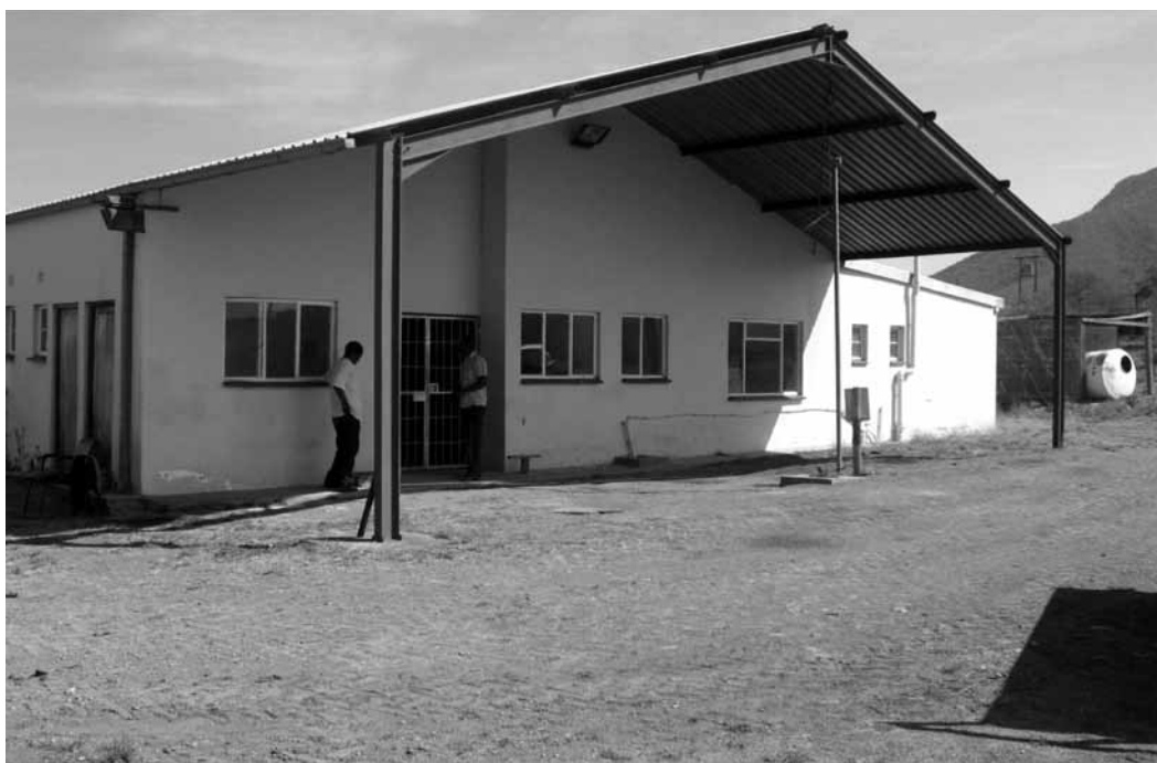
Figure 5.6: Renovated ZIS offices
